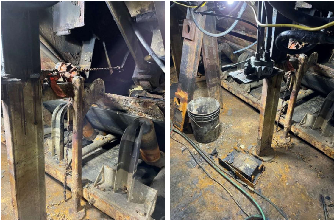
Figure 6. Photographs of Cuyahoga 's portside cargo tunnel at the forward end of gate 22. Source: U.S. Coast Guard.
